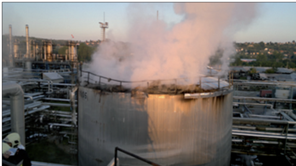
Figure 5: Explosion and fire in bitumen producing factory [14]
