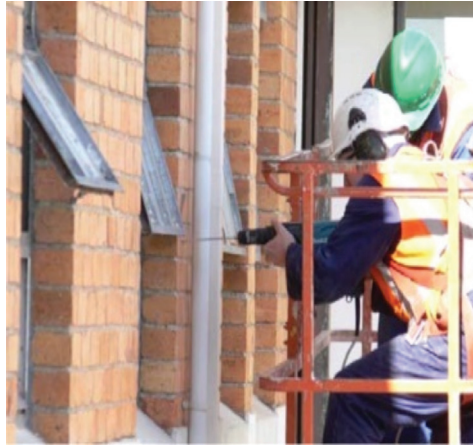
Figure 2. Using steel ties for increasing flexural strength and reinforcing outer structural elements. [19]
