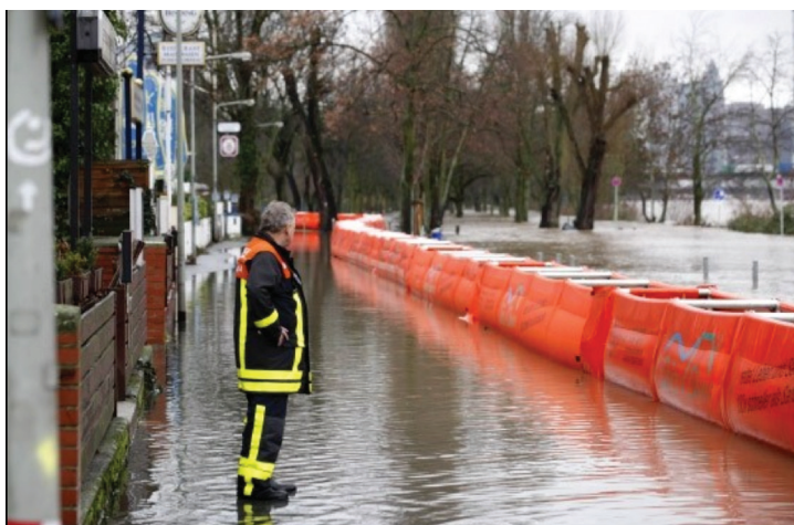
Figure 8. Rapid-deployment mobile dykes. (Made by Dapd, [40])
